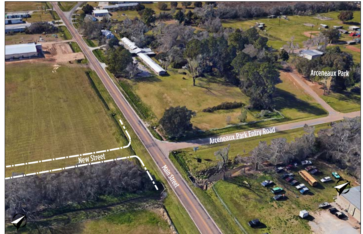
Existing Conditions, Photo Match to Image on Right.
