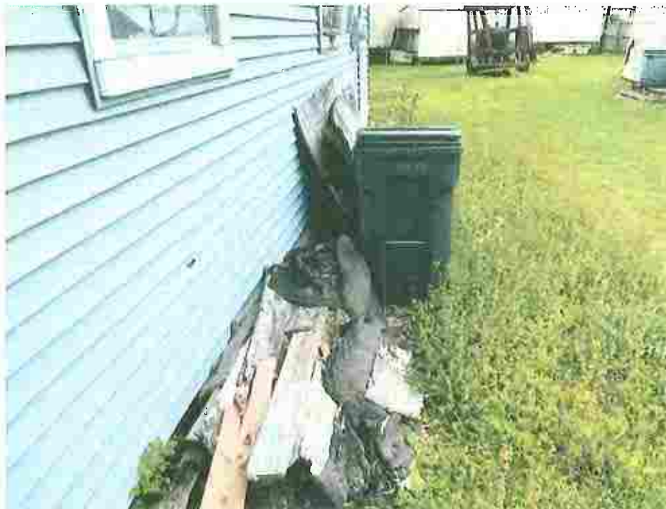
Picture taken April 12, 2023; rubbish and debris piled on property causing blighting and providing habitat for pest and vermin.
